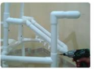
INSERT PUSH PULL HANDLE INTO BACK SECTION AND SECURE USING 1/2" RETAINING SCREWS.
